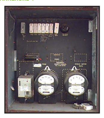
This photograph is an example of an asbestos-based electrical backing board in a typical domestic installation. Note the dust in the bottom of the cabinet and on the fittings. All dusts inside the cabinet are assumed to be contaminated with asbestos.
