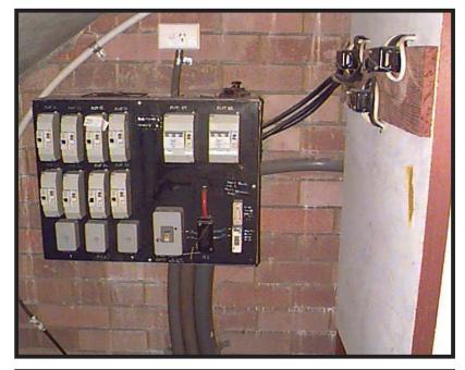
The top photograph shows an asbestos-based electrical backing board inside a cupboard at a commercial premises. The right-hand side of the cupboard is lined with asbestos cement (AC) sheet.
