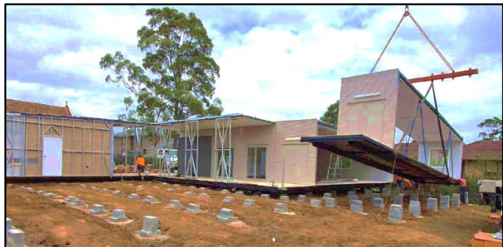
Cranes deliver the Wilton modular church
