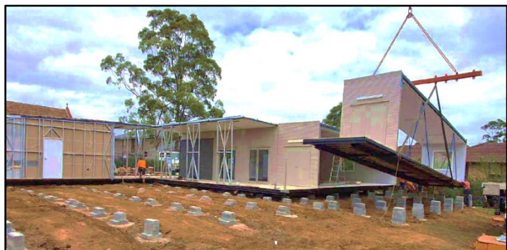
Cranes deliver the Wilton modular church
