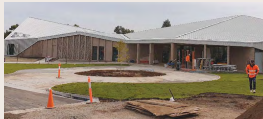
Top to bottom: St Paul's Carlingford redevelopment. Chapter House - St Andrew's Cathedral. New church at Stanhope Gardens.
