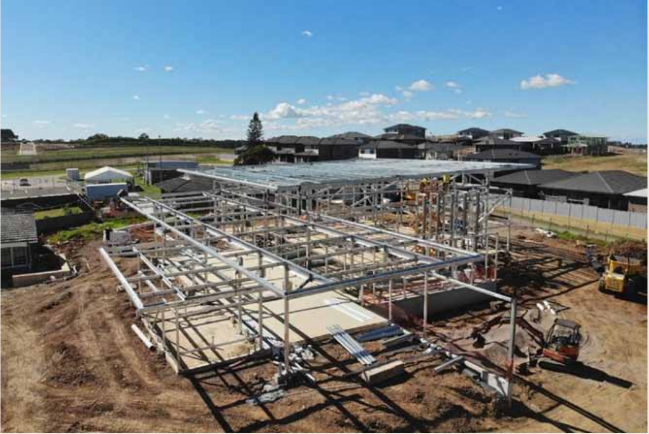
Construction underway at Leppington
