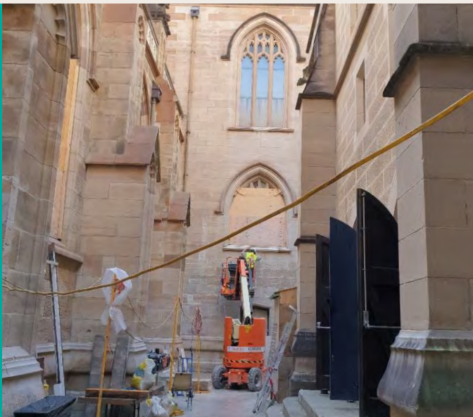
Chapter House exterior works
