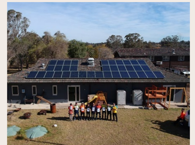
Solar panel installation.
