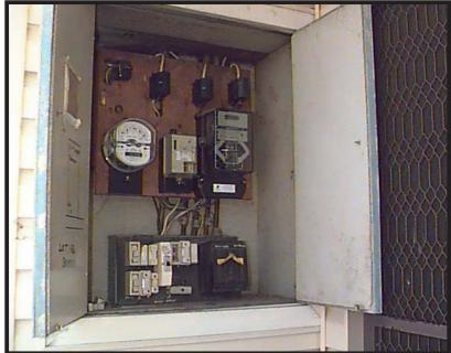
The bottom photograph shows a typical domestic meter box. Although the metering equipment is mounted onto a timber board, the internal faces of the cabinet are lined with asbestos millboard.
