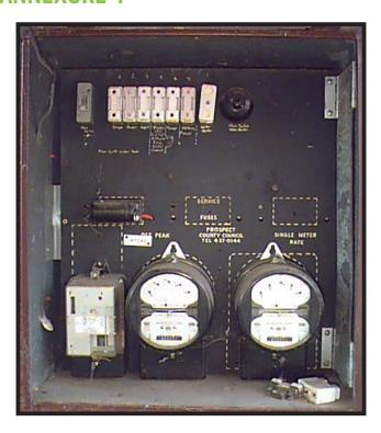
This photograph is an example of an asbestos-based electrical backing board in a typical domestic installation. Note the dust in the bottom of the cabinet and on the fittings. All dusts inside the cabinet are assumed to be contaminated with asbestos.
