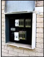
These boards need to have asbestos warning labels attached. This procedure assists in guiding your management of this issue.
