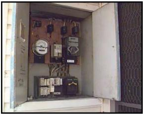
The bottom photograph shows a typical domestic meter box. Although the metering equipment is mounted onto a timber board, the internal faces of the cabinet are lined with asbestos millboard.
