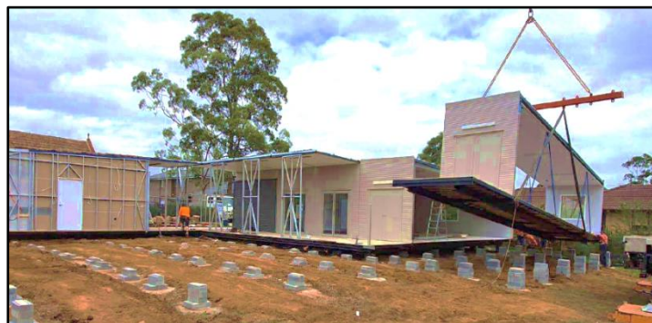
Cranes deliver the Wilton modular church
