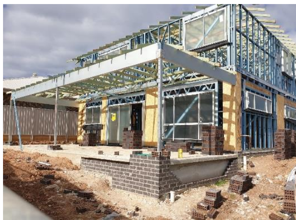
Stanhope rectory under construction
