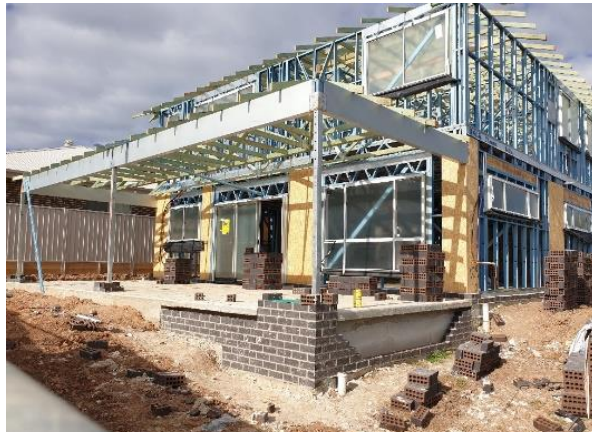
Stanhope rectory under construction
