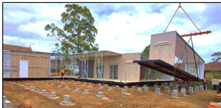
Cranes deliver the Wilton modular church
